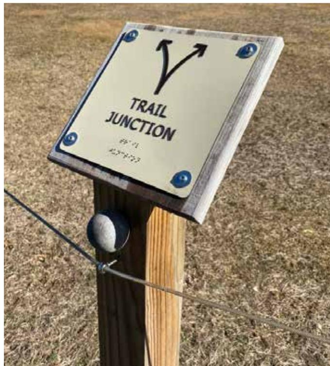
Wayfinding at the Lake Wallace Sensory Trail includes signs in braille connected by a guide wire lining the entire path to provide accessible navigation for those with limited or impaired visibility.
